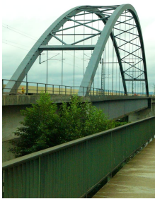
DB Frankfurt: Nets installed
