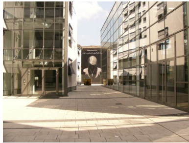
Egana Goldpfeil Offenbach: TAPO electrical system
