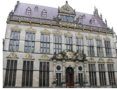
HWK Bremen: Columbox electrical system
